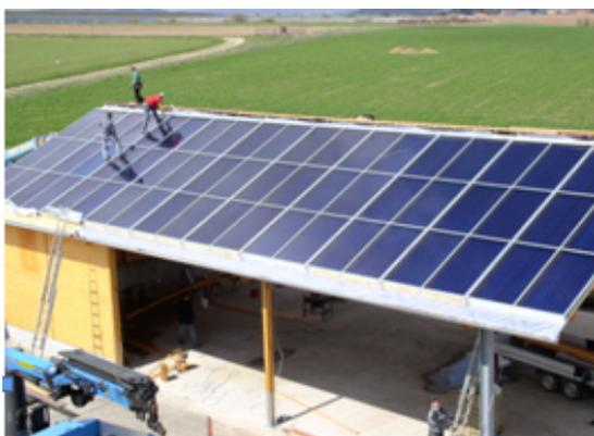
Construction of the solar collector field (155m<sup>2</sup>), April 2012
