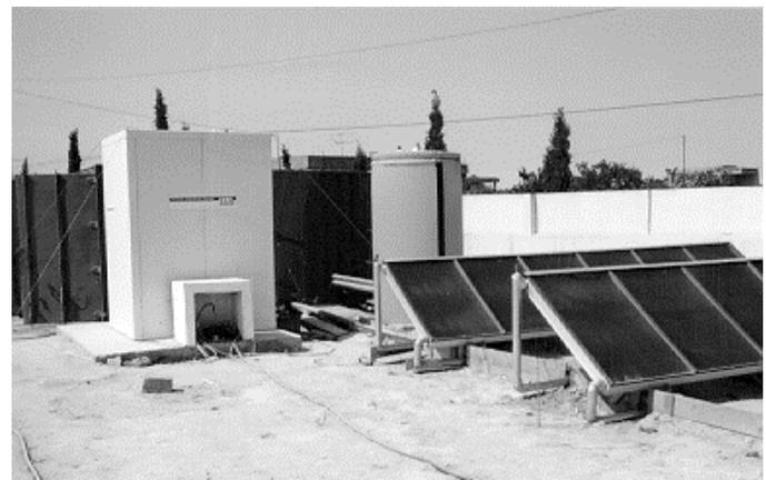
Figure 2: The plant installed in Sfax, consisting of collector, storage and desalination unit
