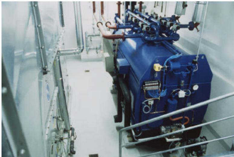
**Figure 5: Mycom adsorption chiller with a cooling capacity of 70 kW, installed at a hospital in Germany.**
