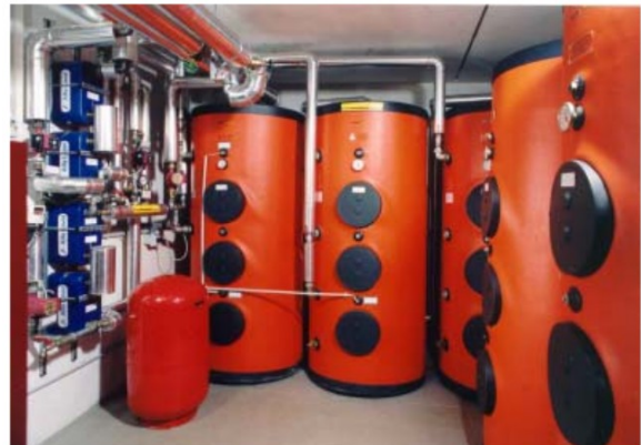
Abb. 1: Speicherkaskade (AEE INTEC 2002)
