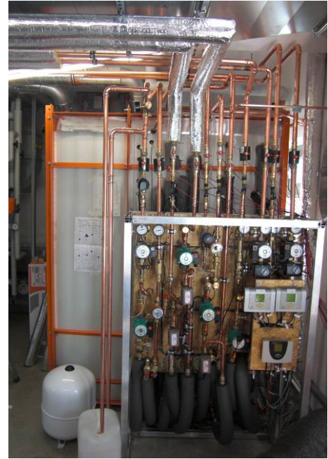
Figure 4. The production hall with a large PV-collector field as well as 30 m 2 of solar thermal collectors (left) and the prototype of the charge and discharge unit in the boiler room (right)
