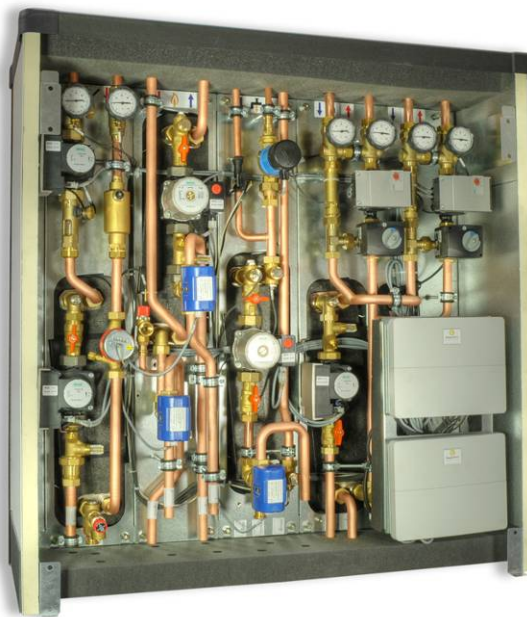
Figure 2. Exhibition model of the charge and discharge unit (without front cover)
